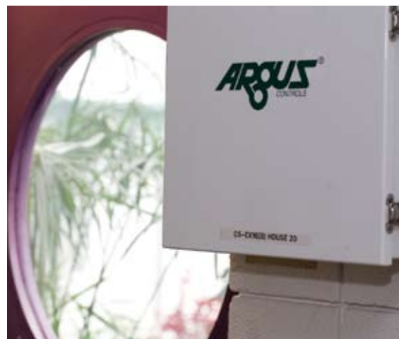
The Argus Greenhouse Control System provides automatic regulation of greenhouse environment and irrigation.
